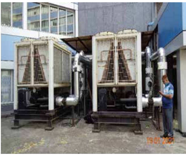
6. Completed Major re insulation work for Blue star Chillers and corroded insulation in Tower A.
