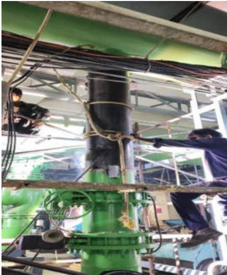
Annual Major maintenance on HVAC piping and valve replacement. Done during Diwali Vacation.
