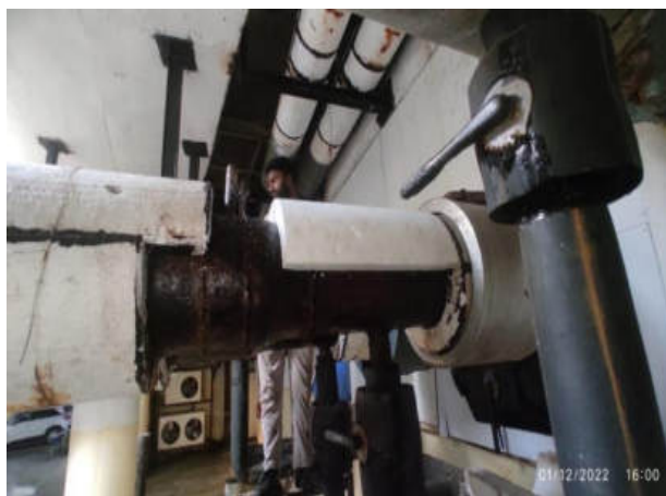
Re insulation of Chill water Header at Upper Basement this will improve the cooling efficiency.
