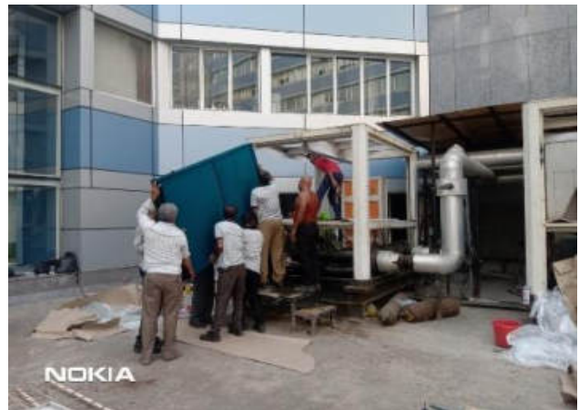
Replacement of old Coils of Standby HVAC chillers at Tower A.
