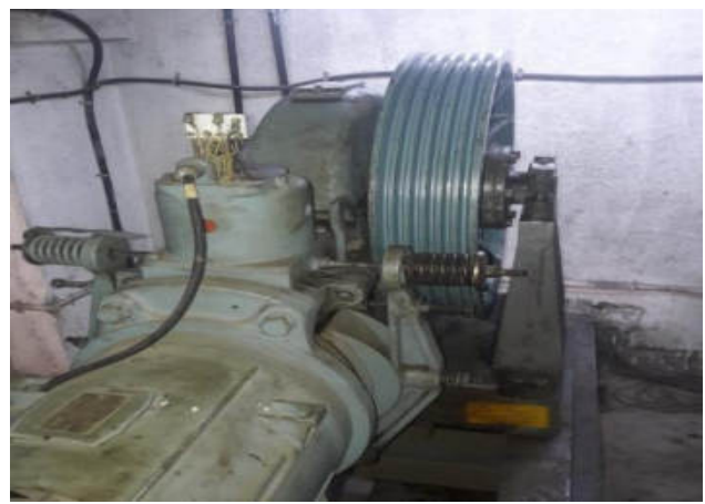
Major replacement of Ropes and Sheaves of Tower elevators to ensure passenger Safety.
