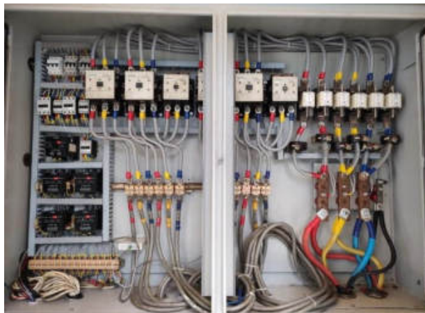
Replacement of Main Control Panel of standby chiller at Tower G.
