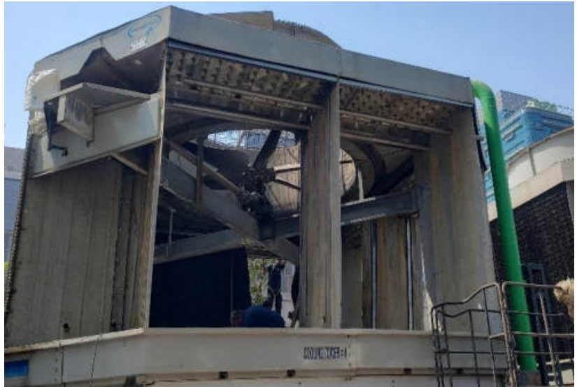
Overhauling and air side part replacement of Cooling towers to keep the equipment ready for summer season.
