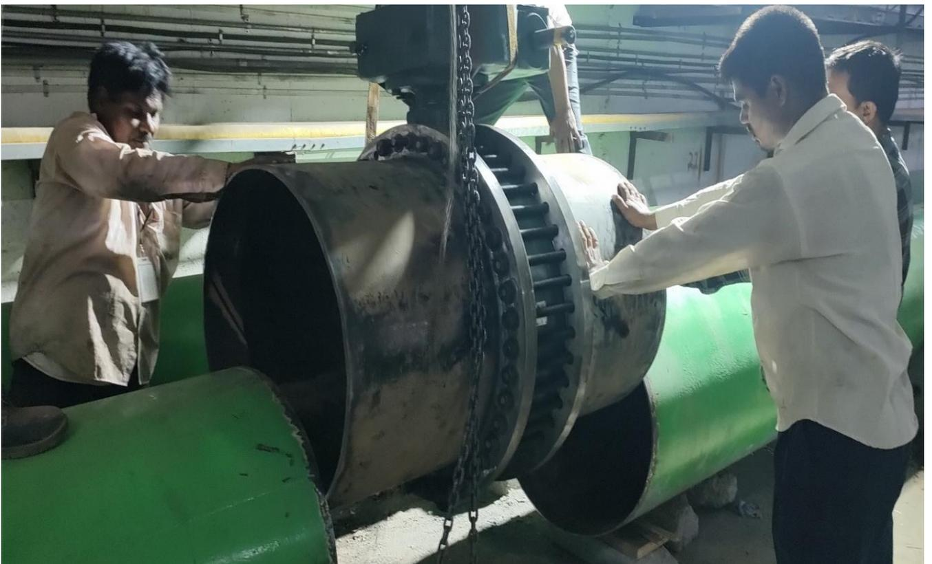
**Major shut down of HVAC system for installation of 4 no's x 750 mm Isolation valve's**
